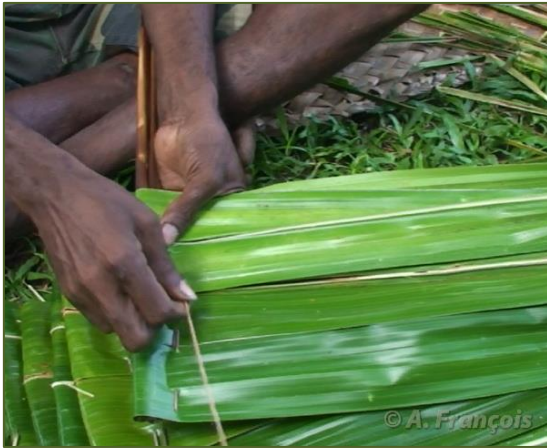
Fig. Pinning the sago leaves ( vēñ no-yot ) for the roof.
