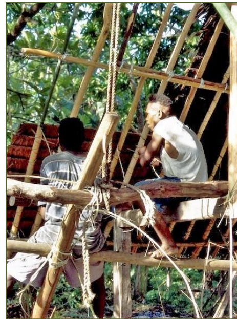
Fig. Thatching the roof with sago leaves ( tigitgiy no-yot ).
