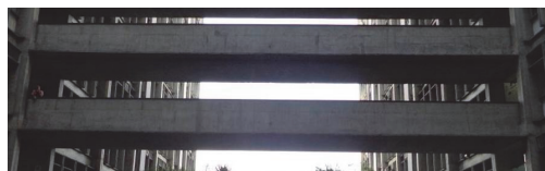
Figure 1. Investigated pedestrian footbridge: lateral view.
