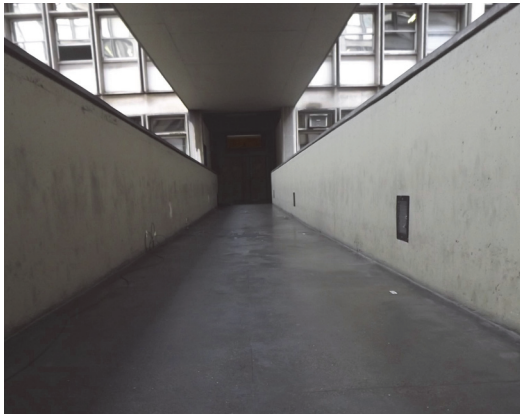
Figure 3. Investigated pedestrian footbridge: front view.
