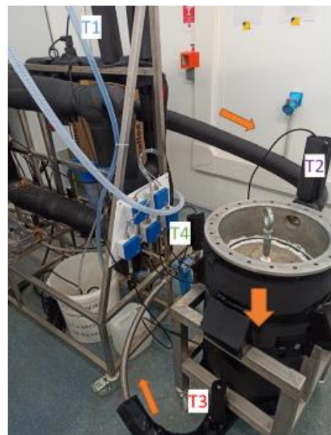
Figure 3. Photo with the distribution of the Pt100/humidity sensors (T1, T2, T3, and T4). The arrows represent the direction of the gas flow. The font colors correspond to the color of the curves in the following figures
