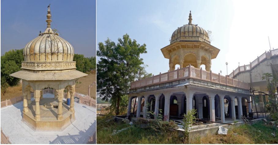
Figure 7. Caraṇa-chatrī of Bhaṭṭāraka Sukhendrakīrti (VS 1886) raised on pillared platform with recently renewed balustrade, next to recent constructions (right on R). Bhaṭṭārakiya Nasiyān, Cākasū, December 2014.
