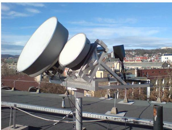
Fig. 3. Antennas and tracking system at BME flat roof.
