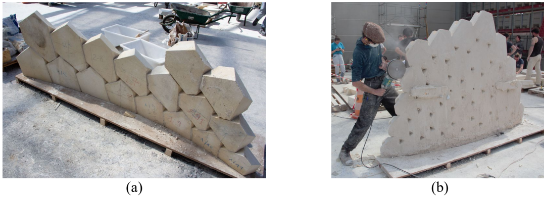
Figure 7: (a) Structure during assembly with plaster and fibers in the joints, (b) preparation of the groove which was filled with fiber and plaster to retain the peripheral blocks
