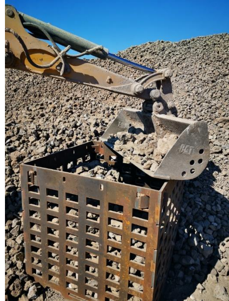
Fig. 1. At left. Structure of the modules studied, without BOF-Slag. At right. Photography of one module filled with BOF-Slag.
