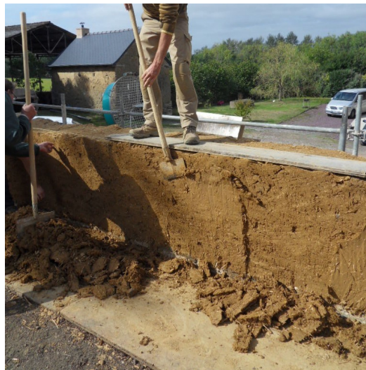
Figure 6. A cob wall in modern construction [33].
