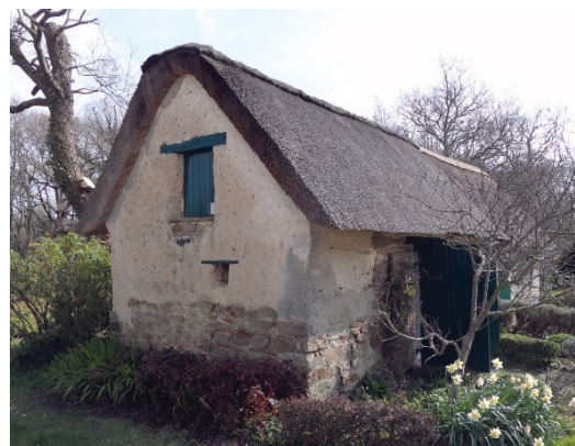
Figure 1. A cob outbuilding at Kerhebé, dating from the mid-19th century [15].
