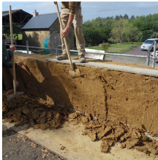
Figure 6. A cob wall in modern construction [33].
