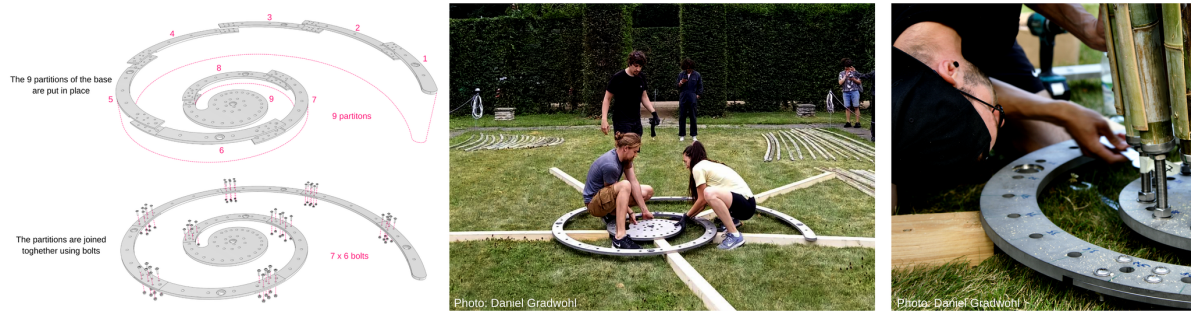
Figure 9: Installing the steel base
