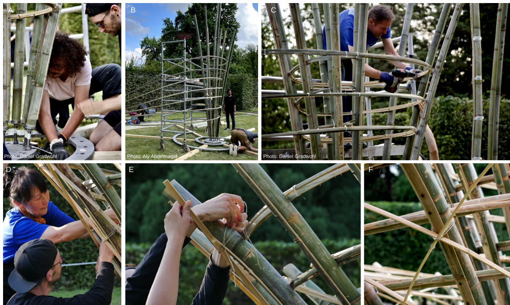
Figure 10: Installing the primary, secondary structural components and the bracing elements
