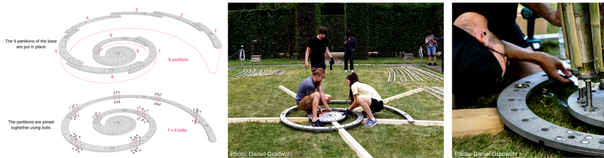
Figure 9: Installing the steel base
