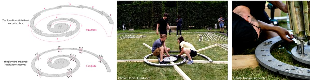
Figure 9: Installing the steel base
