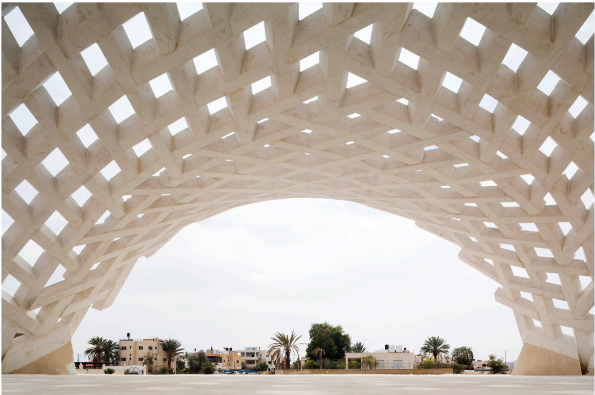
Figure 25: completed structure in Jericho after un-scaffolding
