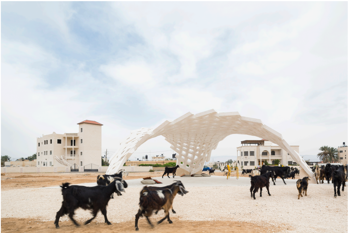
Figure 24: completed structure in Jericho after un-scaffolding
