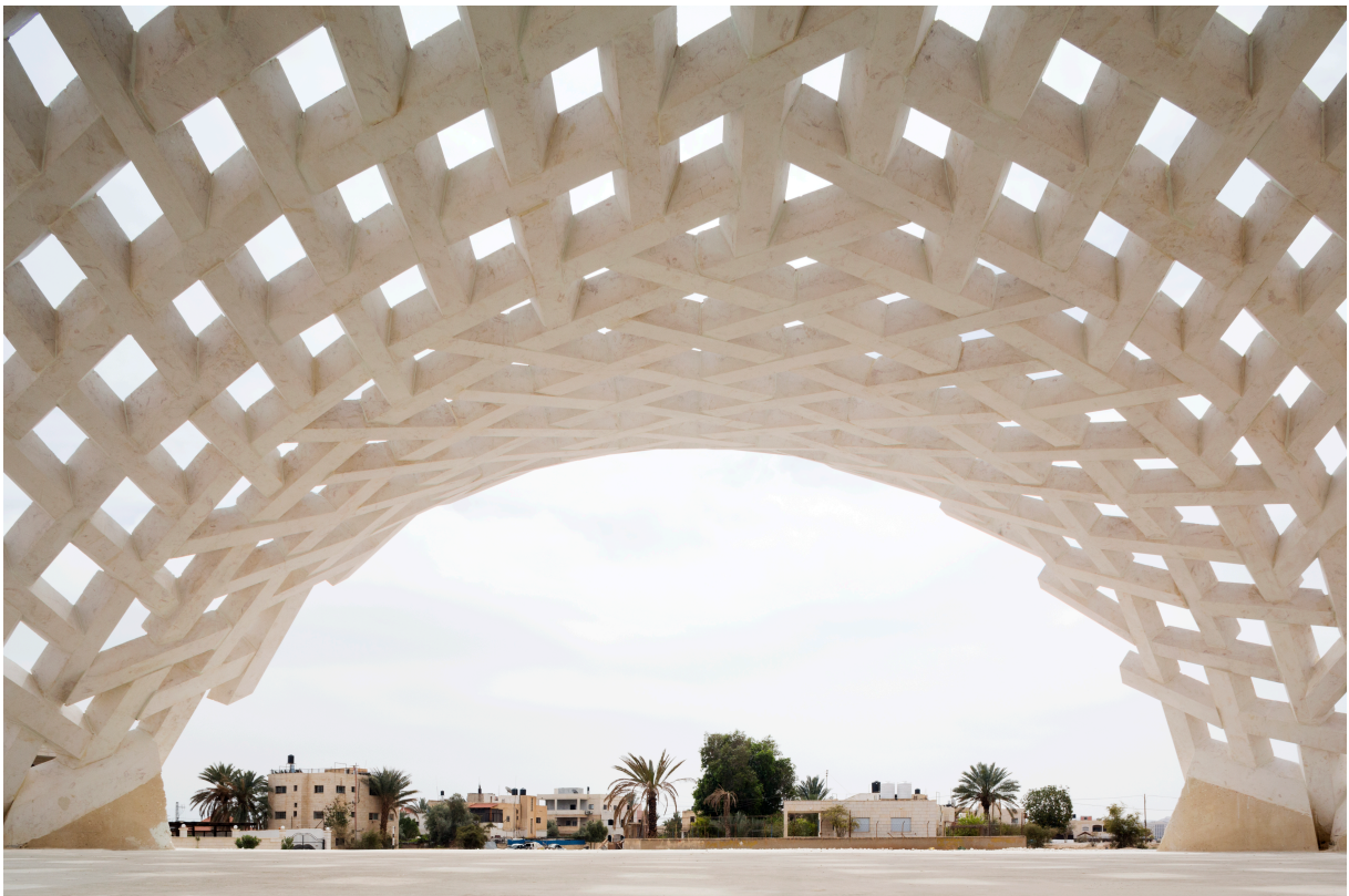
Figure 25: completed structure in Jericho after un-scaffolding
