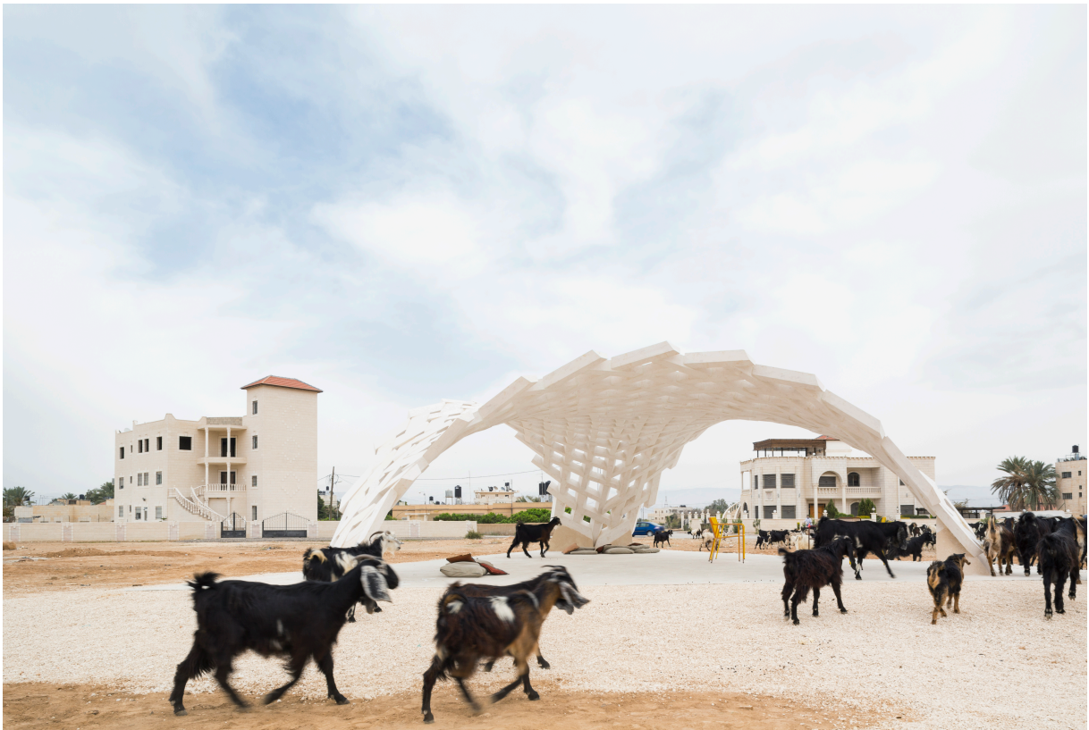
Figure 24: completed structure in Jericho after un-scaffolding
