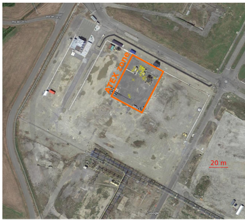
Figure 5. Aerial view of the TADI platform with location of the emission sources (yellow crosses) and the explosive atmosphere area (ATEX zone, depicted as an orange square). Map data: Google, © 2022 Maxar Technologies.
