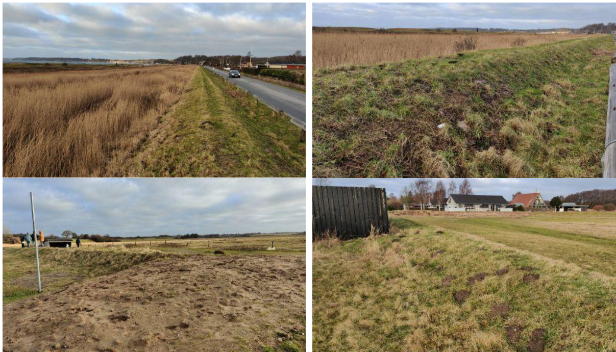
Figure 4: Photo impression of the dike in Hejsager (source: own photos)
