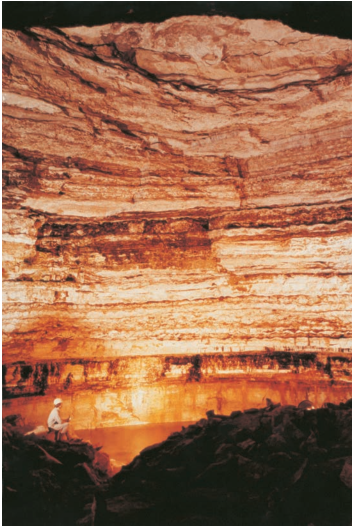
Photo 4: Fontis sous la gare du Nord (Paris 10 e ). Cliché Solétanche, 1975. Sinkhole created by a pocket of dissolution in gypsum (beneath Gare du Nord railway station, 1975). Its stabilisation has necessitated 7,300 m 3 of grouting.
