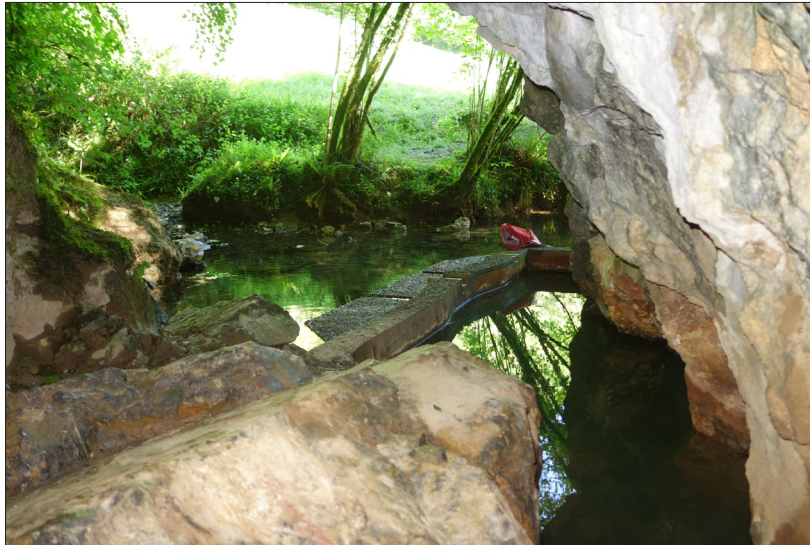
Fig. 1. Inside-out view of the twin springs of Camou. At the beginning of 20th century, a low wall was built to avoid mixing between the cold spring to the left, and the hot spring to the right. A pipe led the water to the nearby farm that was set up as a medical spa (photo. J.-Y. Bigot).
