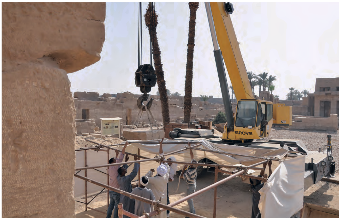
Fig. 5. Removal of the blocks by mean of a crane (E. Saubestre © CNRS - CFEETK).
