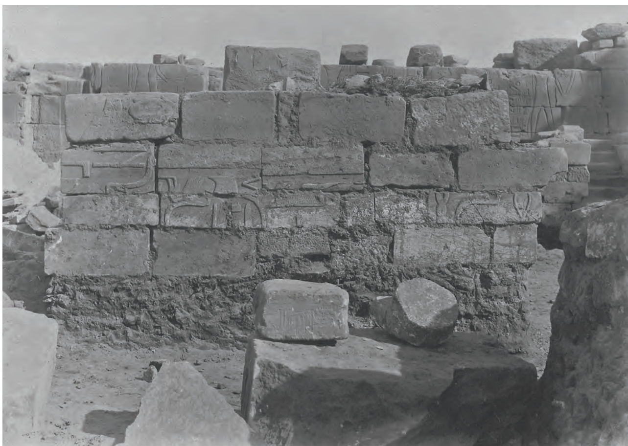
Fig. 30. Remains of the byzantine monastery in the courtyard of the VII th -VIII th pylons, reusing kushite blocks, before their dismantling by M. Pillet. Photo © CNRS-CFEETK, photo n° 68416, archives M. Pillet.
