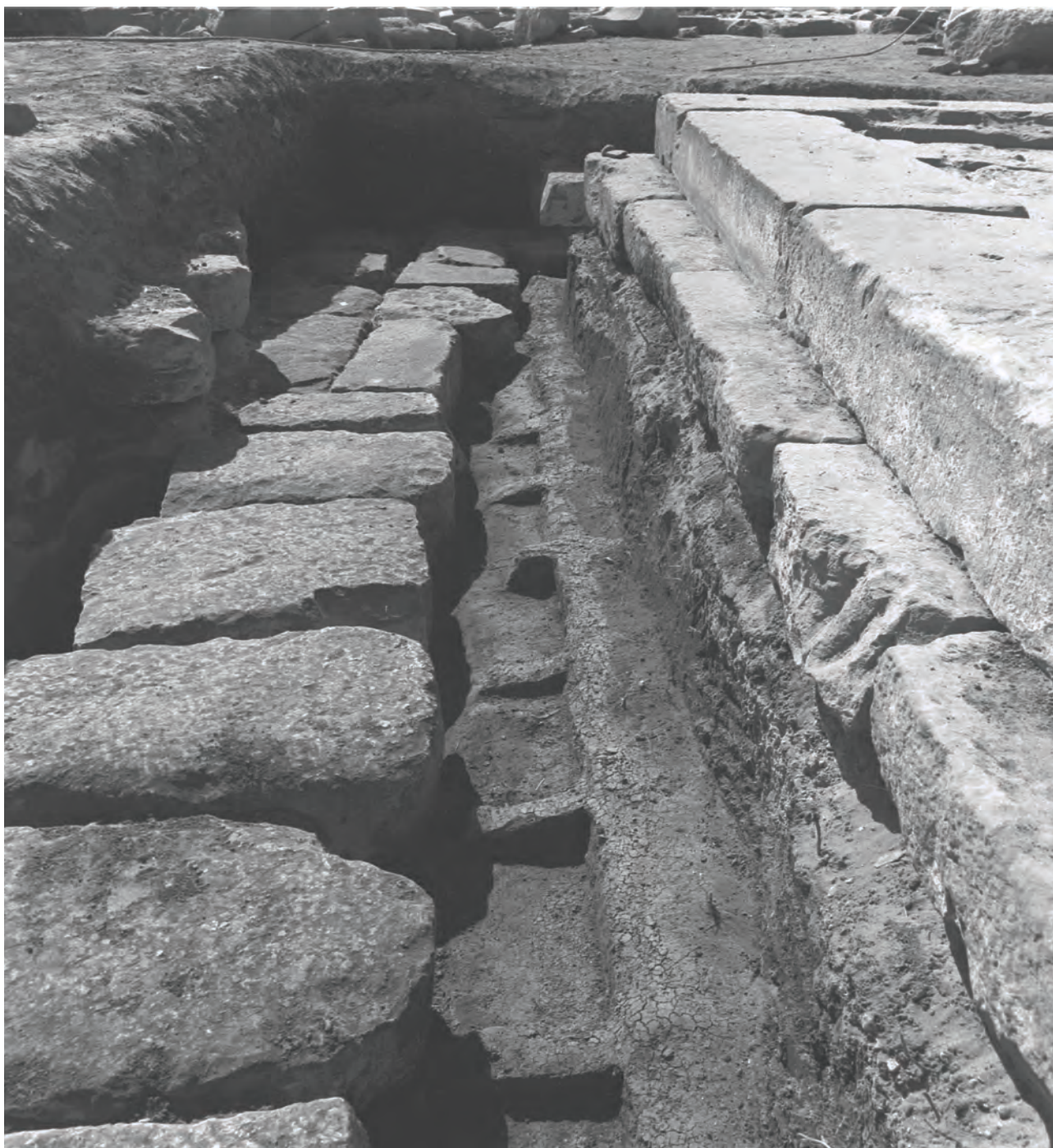
Fig. 22. Eastern part of the mud modelled structure appeared at the level 73,01 between the foundation trench of the sandstone platform and the foundation trench of the limestone substructures (of Senusret I). Photo A. Bellod, © CNRS - CFEETK n° 15588.
