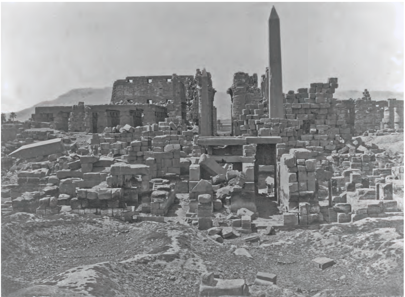
Fig. 35. The Middle Kingdom courtyard on photos of Bonfils ≈ 1870, CFEETK n° 13305.
