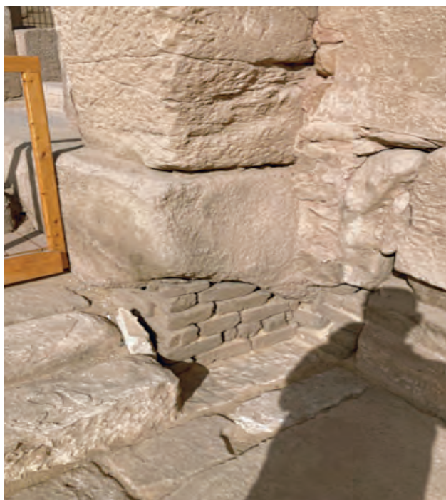
Fig. 31 a-b. The threshold set by Thutmose III which resulted in a L-shape recutting of a limestone channel block which is thus anterior to this king. Thus all the sandstone blocks lying under it are themselves older. (L. Gabolde @ CNRS-CFEETK).
