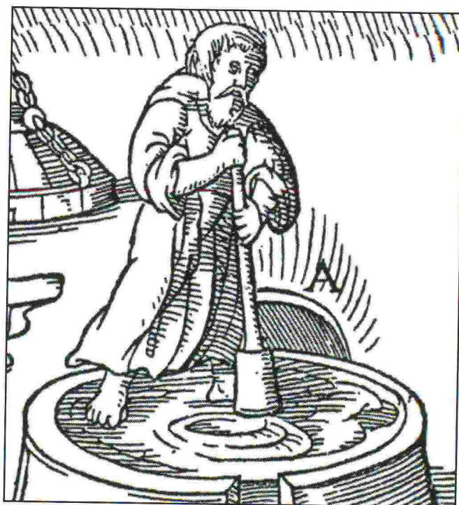
Figure 4: Hearth making illustrated in De re metallica; ash is tamped with a rammer.
