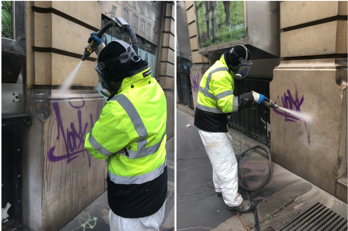
Figure 3. Sandblasting a graffiti (© J. Denis & D. Pontille)
