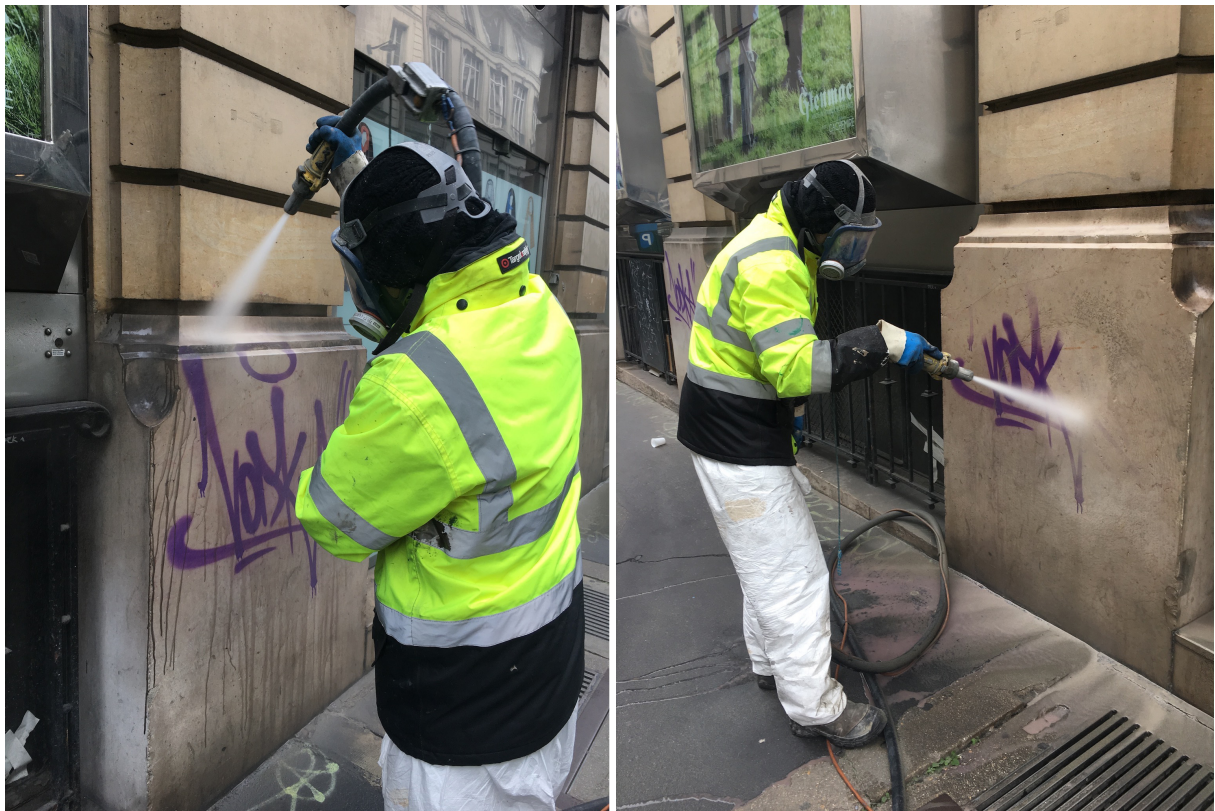
Figure 3. Sandblasting a graffiti (© J. Denis & D. Pontille)
