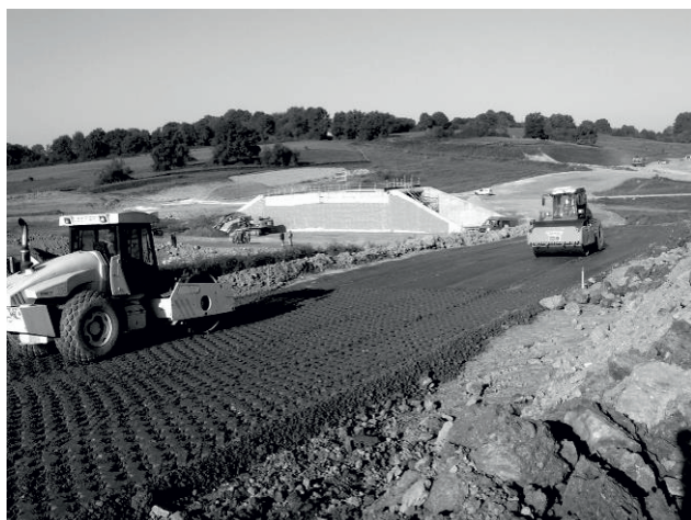
Figure 1. In situ compaction test construction.
