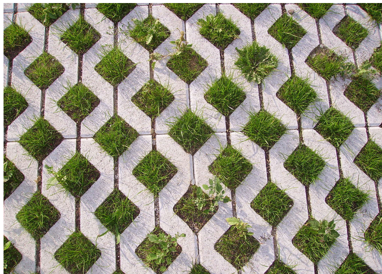
Figure 7: Photograph of a grass paver (credit: I. Giel).
