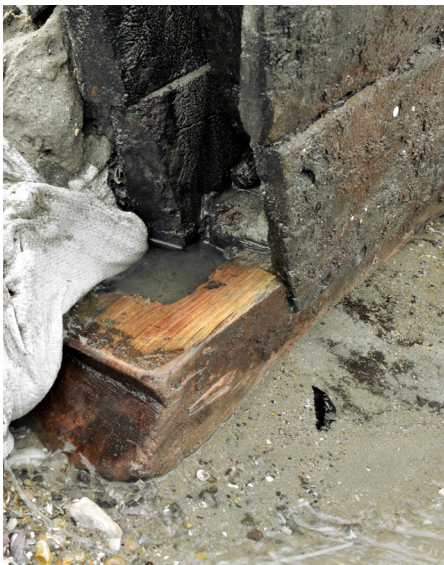
Fig. 1.6. The open mortise in the aft extremity of the keel Source: Images Explorations — F. Osada; E. Rieth/S. Bertoliatti
