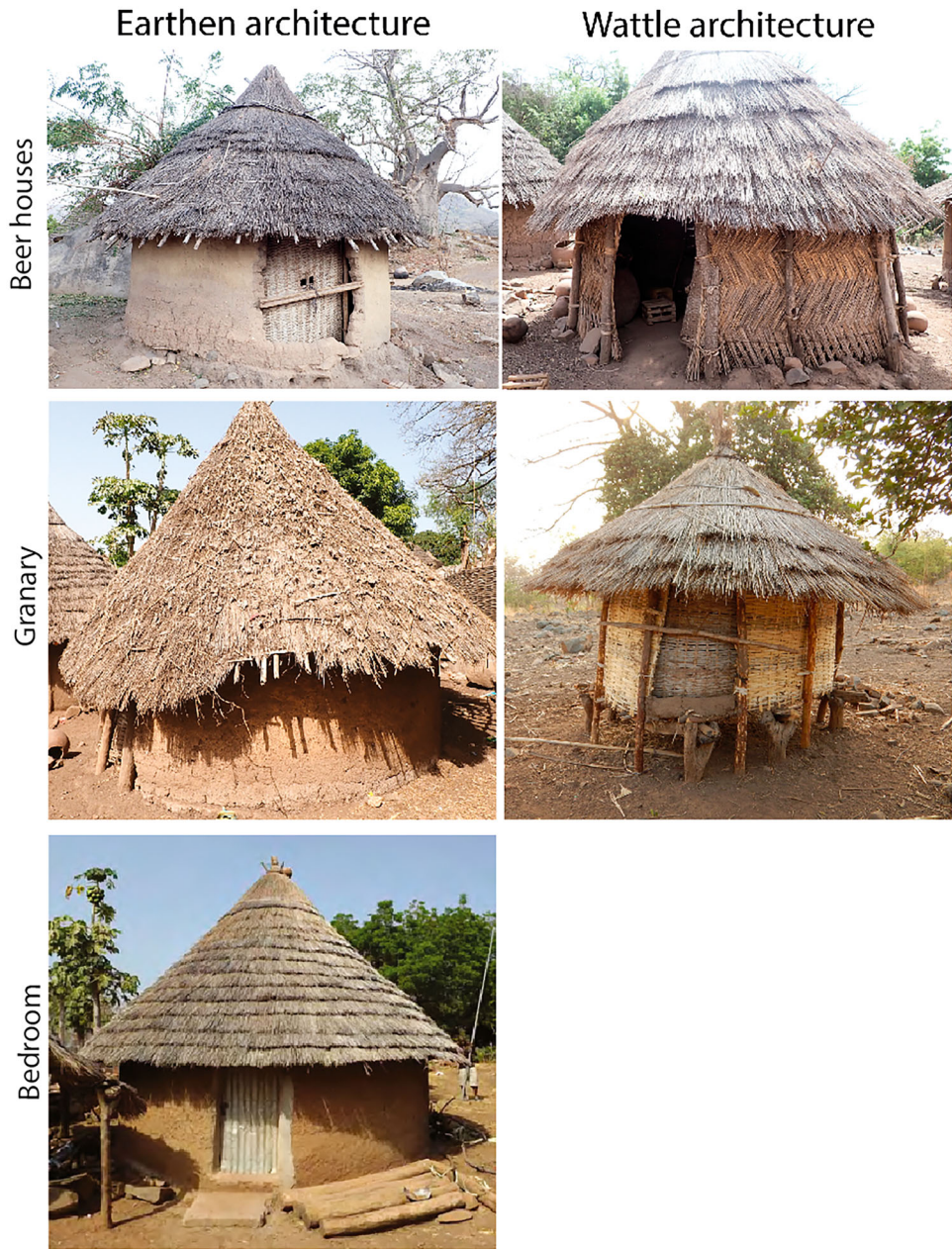
Figure 6. Building materials and techniques of beer houses (top), granaries (middle) and bedroom (bottom).
