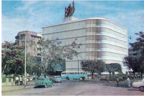
Fig. 48: Mumbai. This rare representation of the Esso building (now Petrol House) shows a projection of the building completed in 1956. The collage technique evokes the practices of the interwar European avant-gardes.
