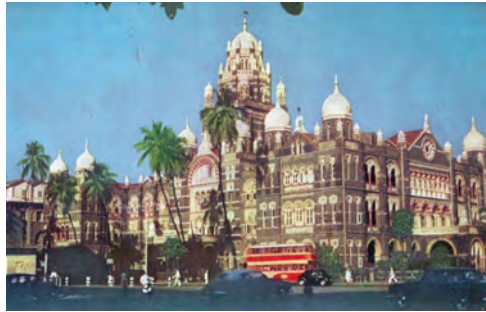
Fig. 35: Mumbai, Western Railway Office.
