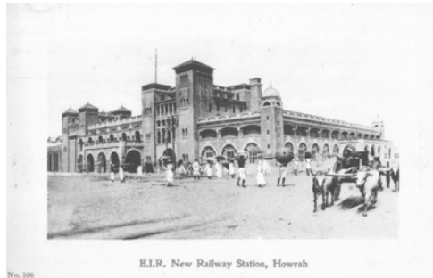
Fig. 33: Howrah, New Railway Station.
