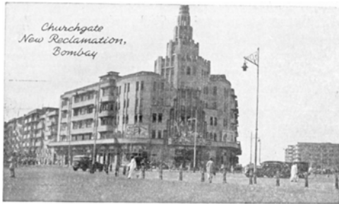
Fig. 2: Eros Cinema (1938): an Art Deco-style monument built by Indian architects but furnished with lifts from Stigler (Italy).
