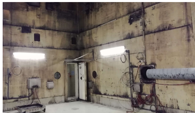
Fig. 12 The 400 m 3 volume of the confined and mechanically-ventilated PLUTON facility.
