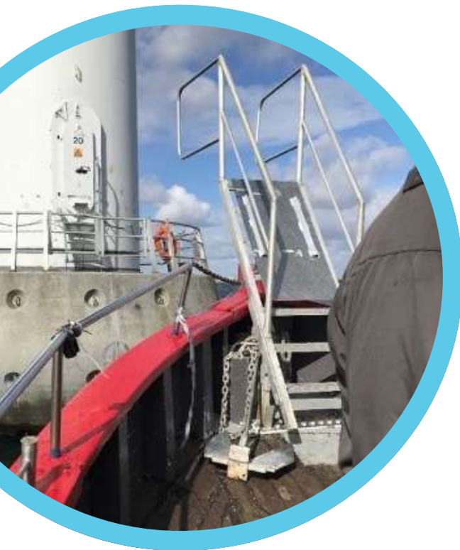
Access to the Middelgrunden turbine with a boat showcasing the ladder system in use.
