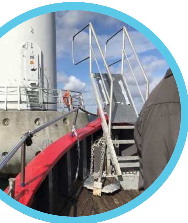
Access to the Middelgrunden turbine with a boat showcasing the ladder system in use.
