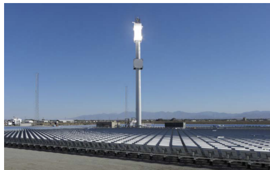
Figure 12: The study case is the eSolar's modular CSP plant in Lancaster. Lines of heliostats are installed to reflect solar irradiance to the central receiver, which is brightened in the figure. Each mirror corresponds to a point in each sub-figure of Fig.13. Tis image is reproduced from Zavodny et al. (2015) with permission from "Elsevier".
