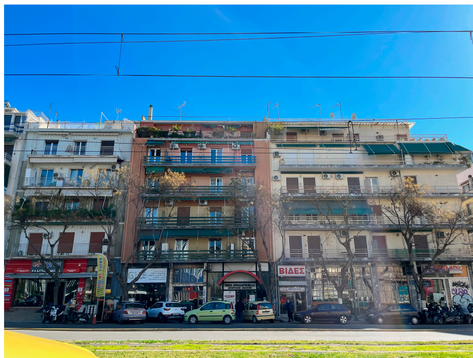
Figure 6. Apartment buildings in vertically segregated neighborhoods in Athens. Photo by authors.
