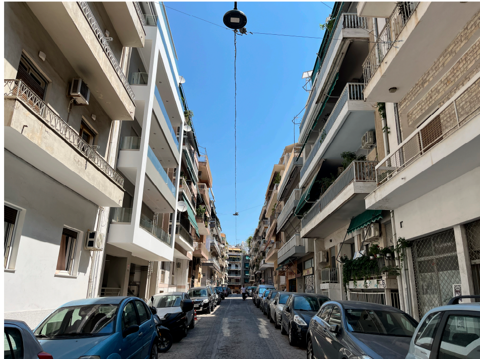
Figure 7. Apartment buildings in densely built vertically segregated neighborhoods in Athens. Photo by authors.
