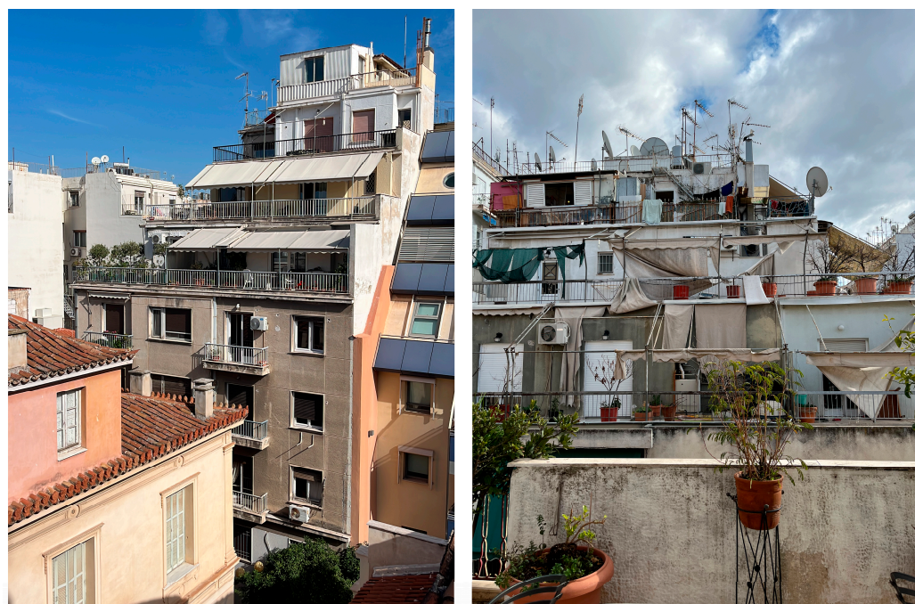
Figure 8. Upper floors and doma rooms in apartment buildings. Vertically advantaged areas (left) and vertically disadvantaged areas (right). Photos by authors.
