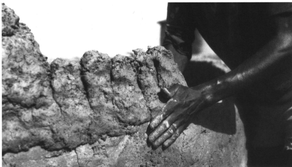
Fig. 4: Squeezing the banco as the lumps are placed in a row, and compressing the new row against the preceding layer (Esapu, March 1989).
