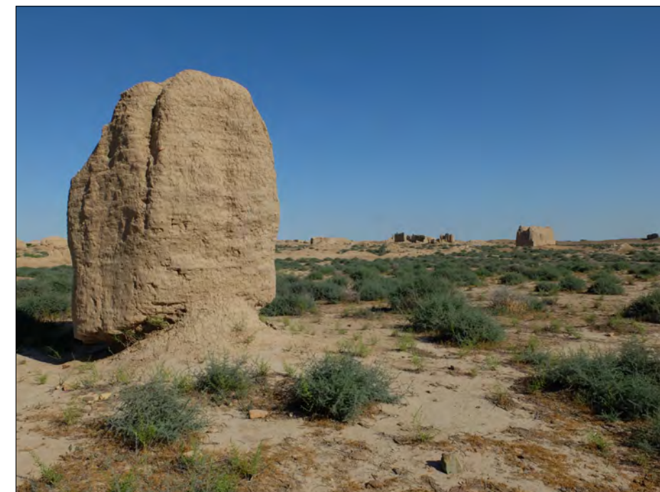
Figure 10. Undercut pathology in Ancient Merv (Turkmenistan) ©CRAterre_C. Sadozai 2015
