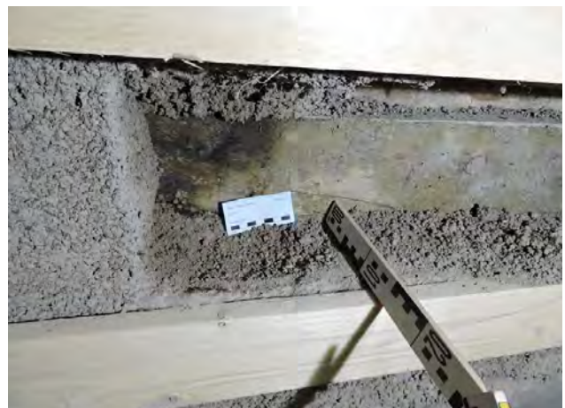
Fig. 4a and b Mould and fungi development because of a too slowly drying processof the light earth interior insulation, Germany
