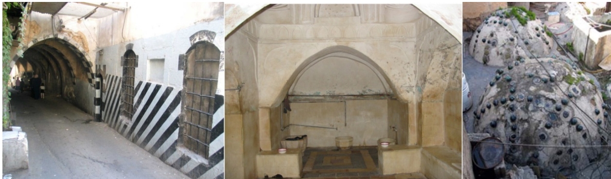
Figure2: Interior and exterior parts of the hammam before restoration (Author, 2007)
