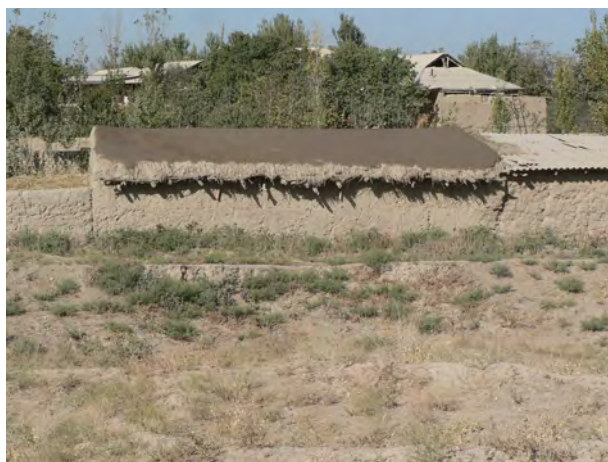
Fig 7: Barn flat roof covered with a special clay, Avazali 2012. Photo : D. Gandreau
