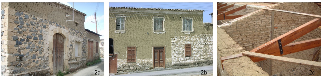
Fig.2. Adobes used in vernacular (2a, 2b) and contemporary architecture (2c)
