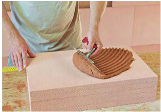
Fig. 3a and b interior insulation with soft fibreboards (a) and mineral foam pannels (b) embedded in earthen mortar
