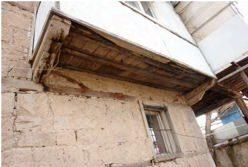
Fig. 6 Special blocks have been made, which could simply move horizontally in case of seismic activity.
