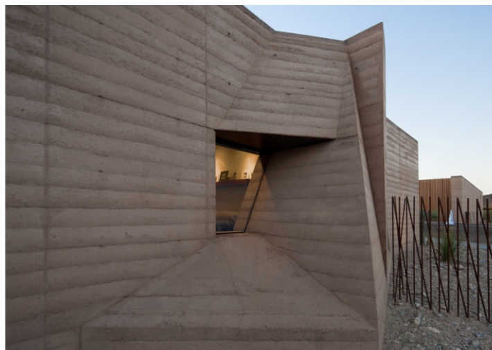
Fig.8 – Outpost House, Paradise Valley, Arizona, USA (Credits: Eddie Jones)
