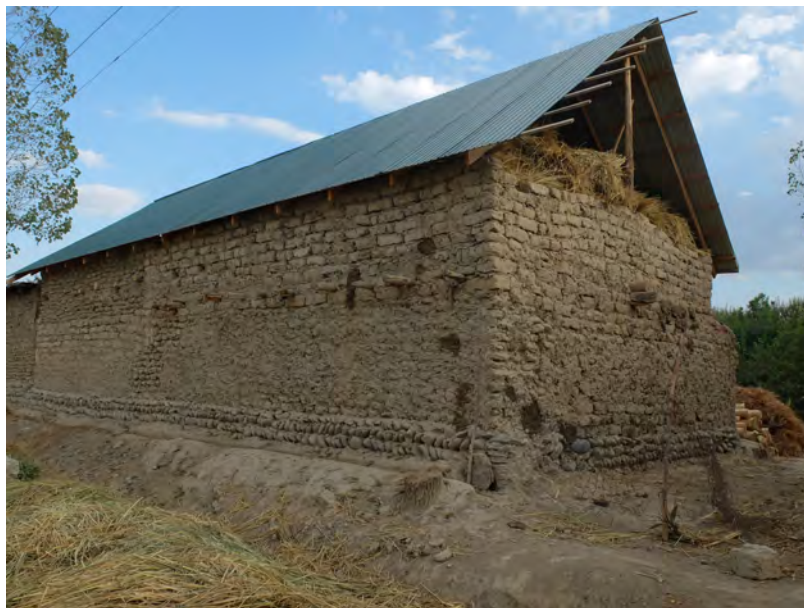
Fig 4: Pebble socle, adobe and hand-molded cob, Avazali 2015. Photo : C. Sadozai
