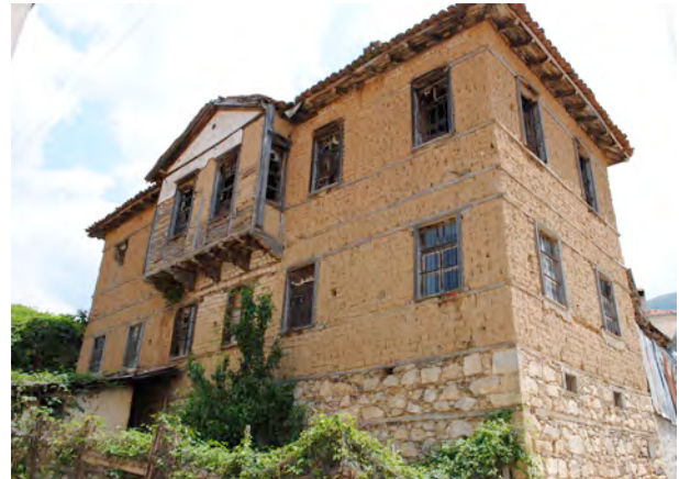
Fig. 7 - House with a projection of the central space and pediment in Antartiko, Prespes.
