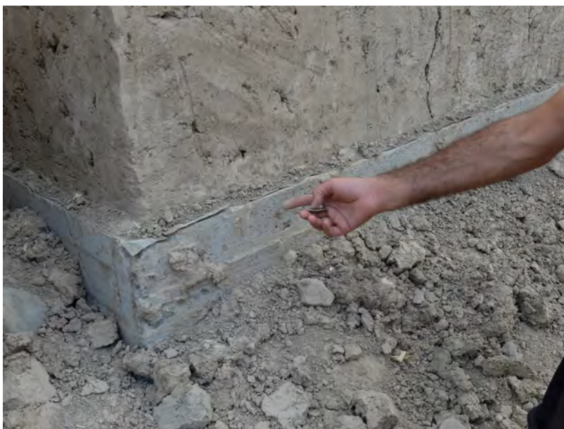
Fig 5: Concrete socle and bitumen fabric, Avazali 2015. Photo : C. Sadozai
