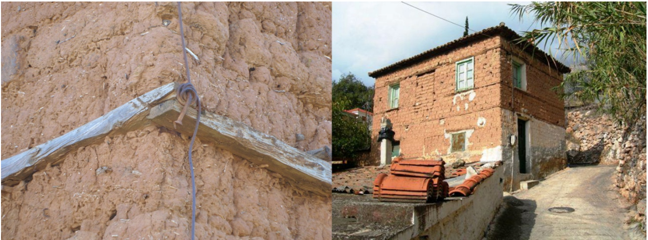
Fig.3 _ An example of horizontal wall tie on an earthen Greek house: the «klapes».
