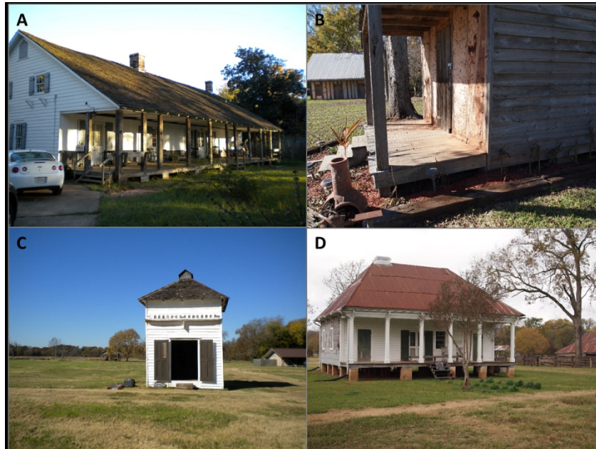
Figure 3. A large variety of Louisiana property types are constructed using bousillage.
