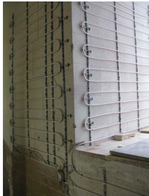
Fig. 6a and b internal insulation of mineral foam pannels (embedded and plastered with clay) and wall heating system at a granary in Freiberg / Saxony in Germany
