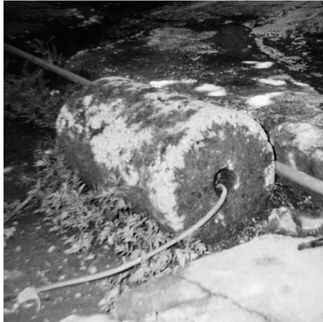
Fig. 7 Cylindrical stone for ramming called <<logh>>
