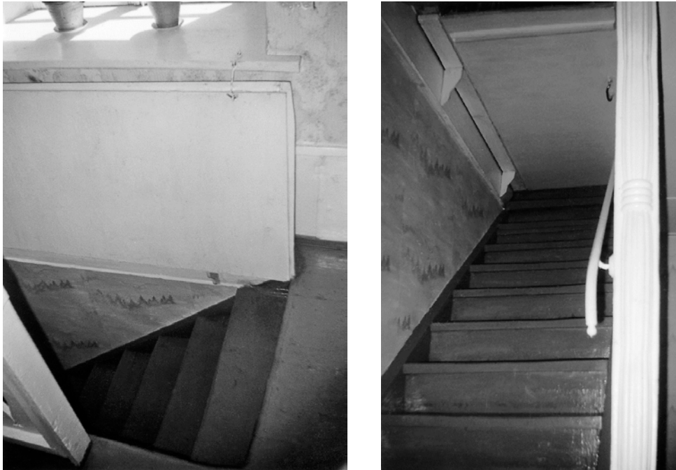
Fig. 9 Staircases pore with the wooden cover <<gabanq>>
