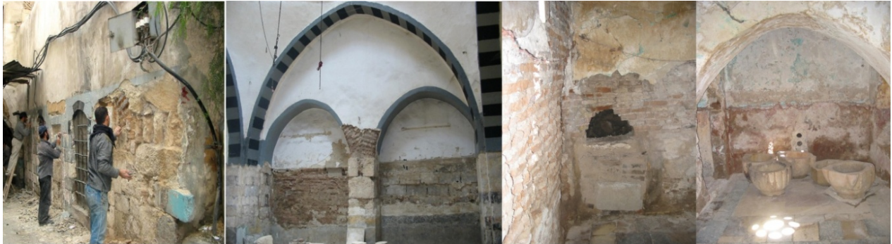
Figure 3: Cleaning phase, removing all types of coating (Author, 2007)
