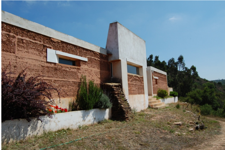
Fig.3 – Troviscais House, Odemira, Portugal (Credits: Marques, 2014)
