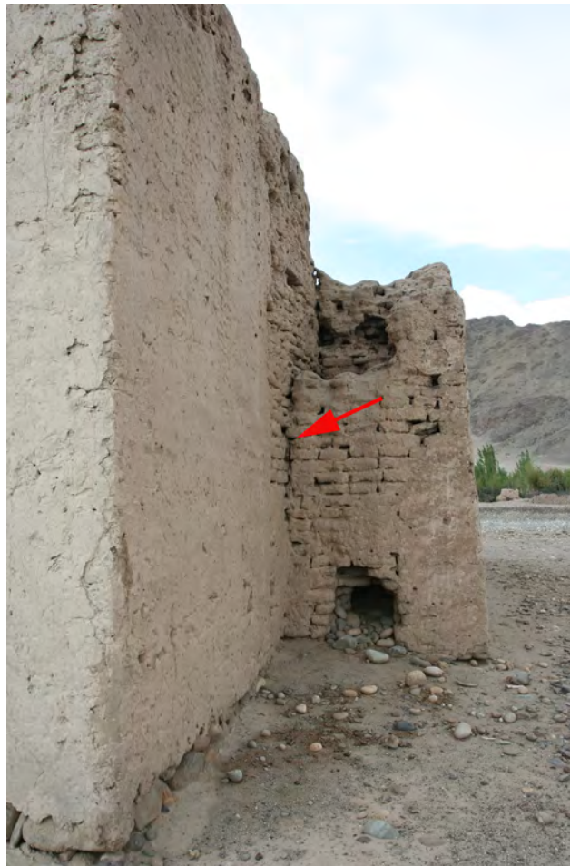
Fig. 10 Temple IV. Side niche without a brick bond to the adjoining cella structure.
