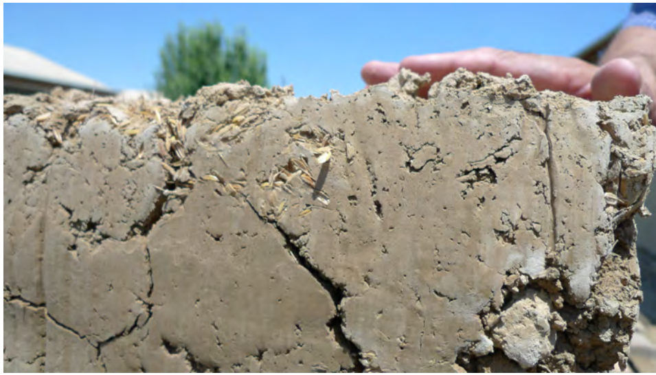
Fig 3: Detail of rice glume in pakhsa, Avazali 2012. Photo : D. Gandreau
