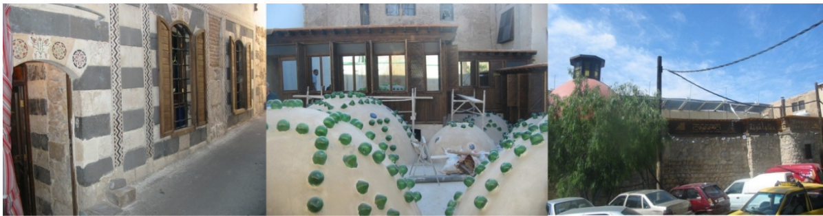
Figure 8: External walls and the roof after restoration (Author, 2010)
