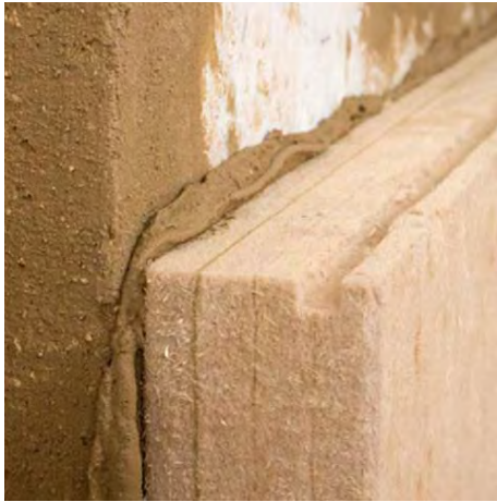
Fig. 3a and b interior insulation with soft fibreboards (a) and mineral foam pannels (b) embedded in earthen mortar
