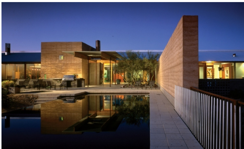
Fig.4 – Low Compound House, Scottsdale, Arizona, USA (Credits: Eddie Jones, 1997)
