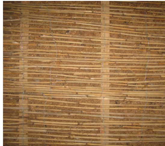
Fig. 5a and b light earth interior insulation with hemp. Former sheepfold Ribbeck / Germany
