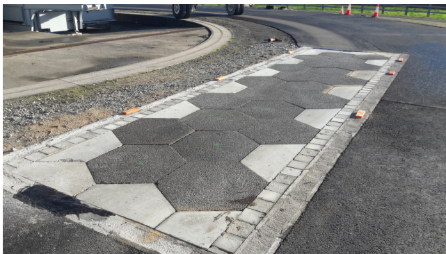
Figure 2: RUP test site.
