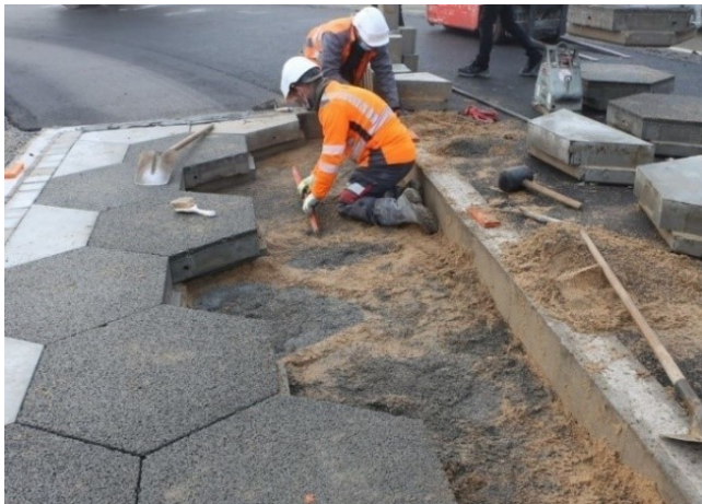
Figure 4: Construction of the test structure at Gustave Eiffel University.
