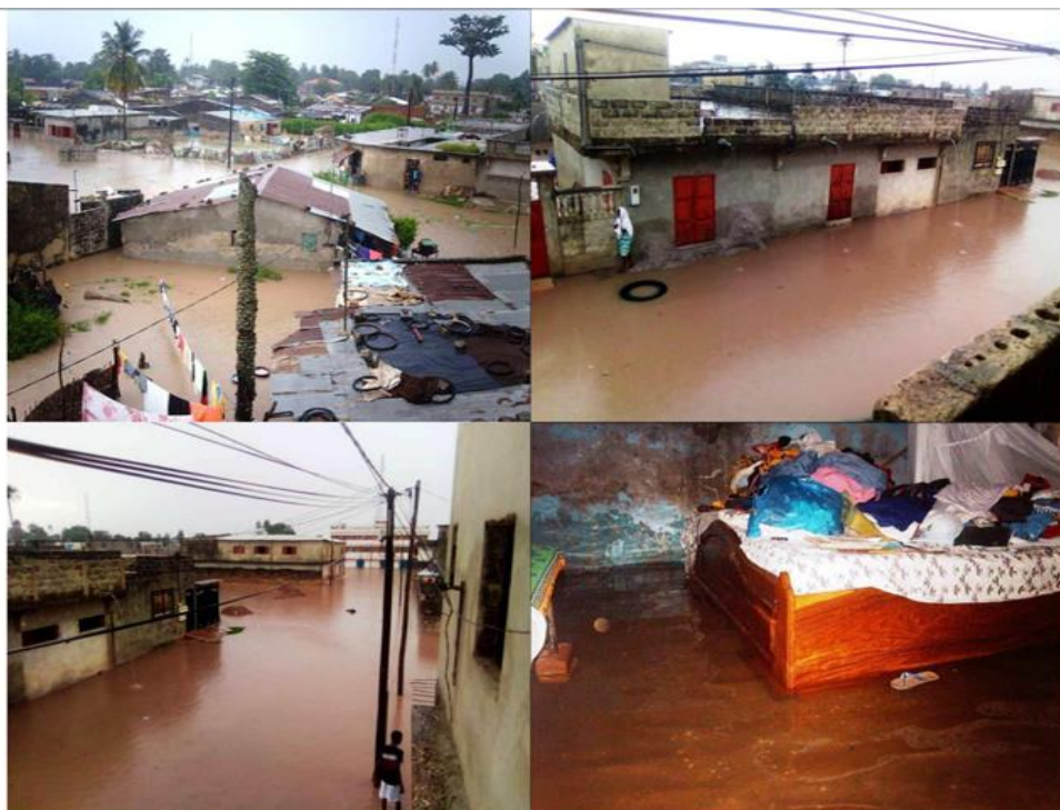
Figure 3. Flooded neighbourhoods in Boudody, Lindiane, Goumel and Belfort (Source: Gomis, 2021)
