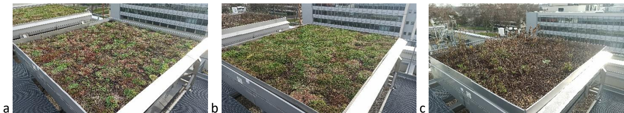
Figure 3. Photos of a) Stromboli - 60 mm substrate, b) Monstro - 120 mm substrate, and c) Gedeon - 240 mm substrate under installation phase with naturally grown vegetation before upper trays with sedums are installed (January 2023).
