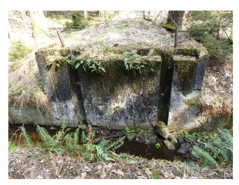
During the 1930's and the construction of the Maginot Line, the water resources of the ponds in the Rothenbach and Schwarzbach valleys were mobilized to create a water cut by flooding the valley. A system of gates and thresholds structured the flood zone and was intended prevent flooding.
