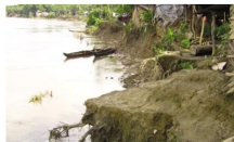
River Bank Erosion after Flood in Bangladesh. Source: CNRS, Dhaka.
