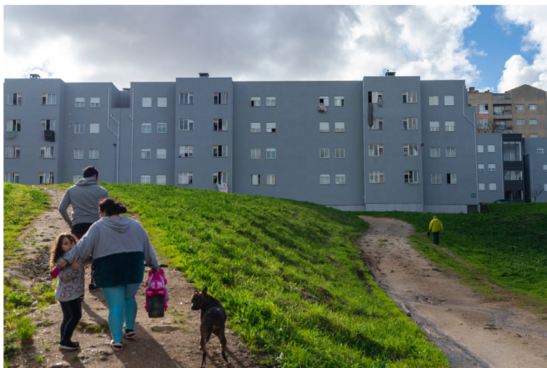
Fig. 1 Accessibility to social housing neighborhoods, Falcão Neighbourhood, Campanhã, Porto. Photo by Carlos Barradas.
