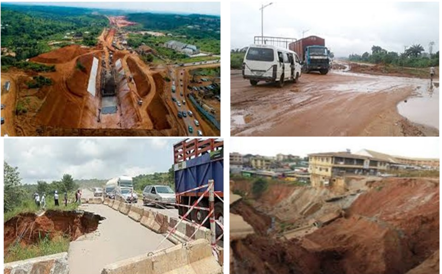
Figure 7: Typical erosion sites in Onuiyi-Nsukka, Udi, Enugu state (Source: News agency of Nigeria, 2011)
