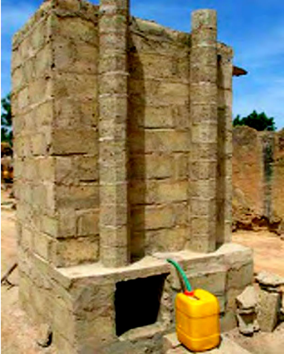
Figure 2. Urine diversion for a compost toilet (Photo by Karin Ahlgren, used with permission) (Kvarnstrom et al., 2006: 7) Source: Ray (2010)
