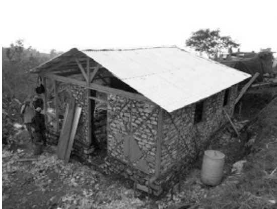
Figure 1: Traditional Haitian timber-frame house
