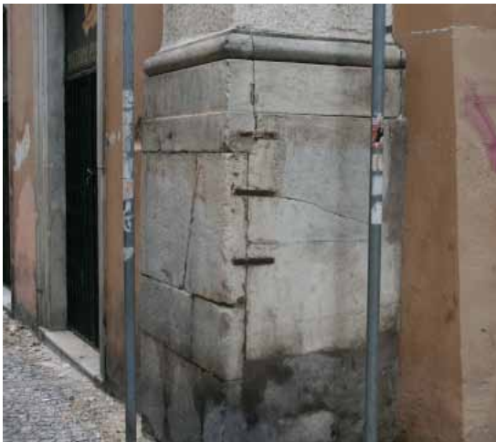
Figure 18a : the 17th century building's pillar repair (POURSOULIS, 2009a)
