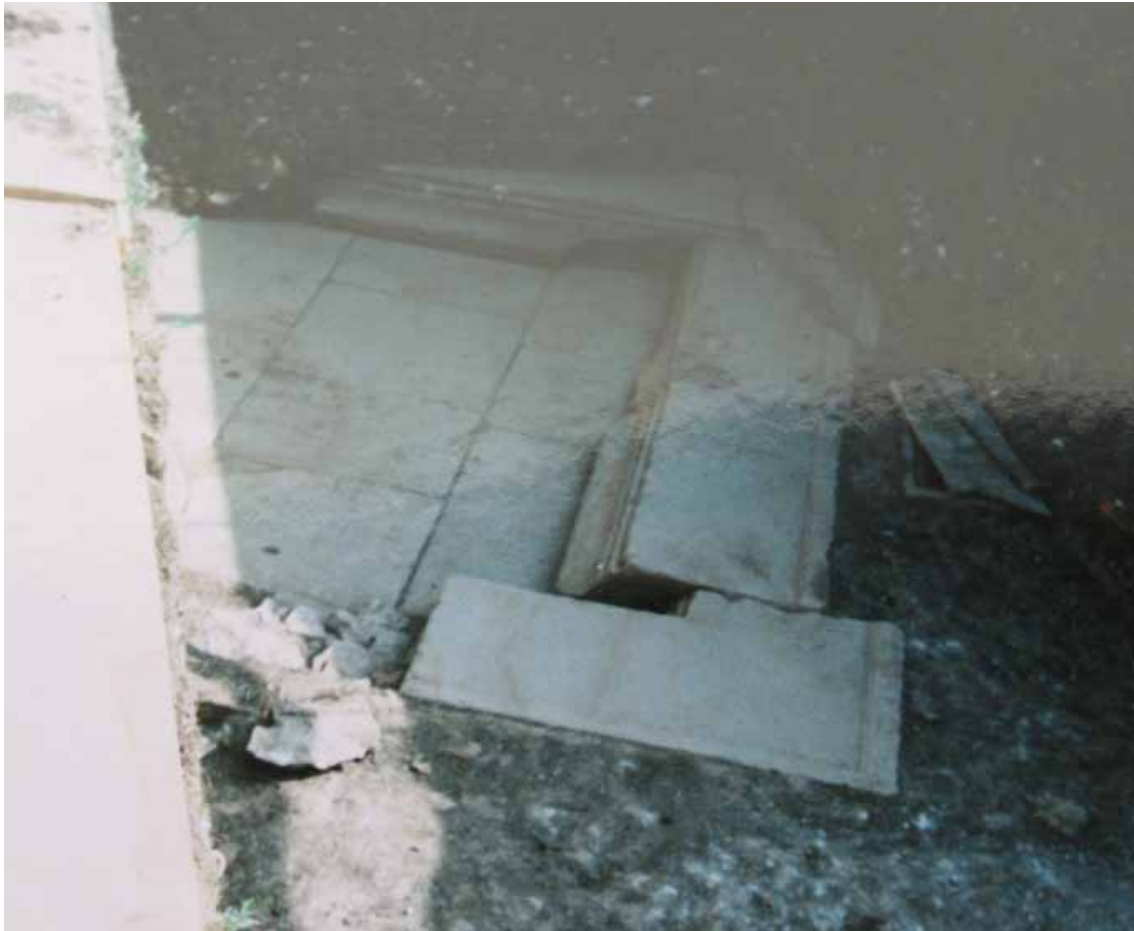
Figure 20: broken pavement in Amiternum villa (archaeological excavation, POUSSOULIS, 2008)
