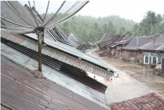
Figure 16: Metal roof coverings in Hilinawalö Fau
