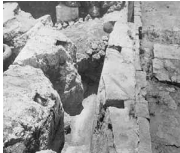
Figure 9b : double facing wall tied with wood beams at Knossos Palace (EVANS, 1928)
