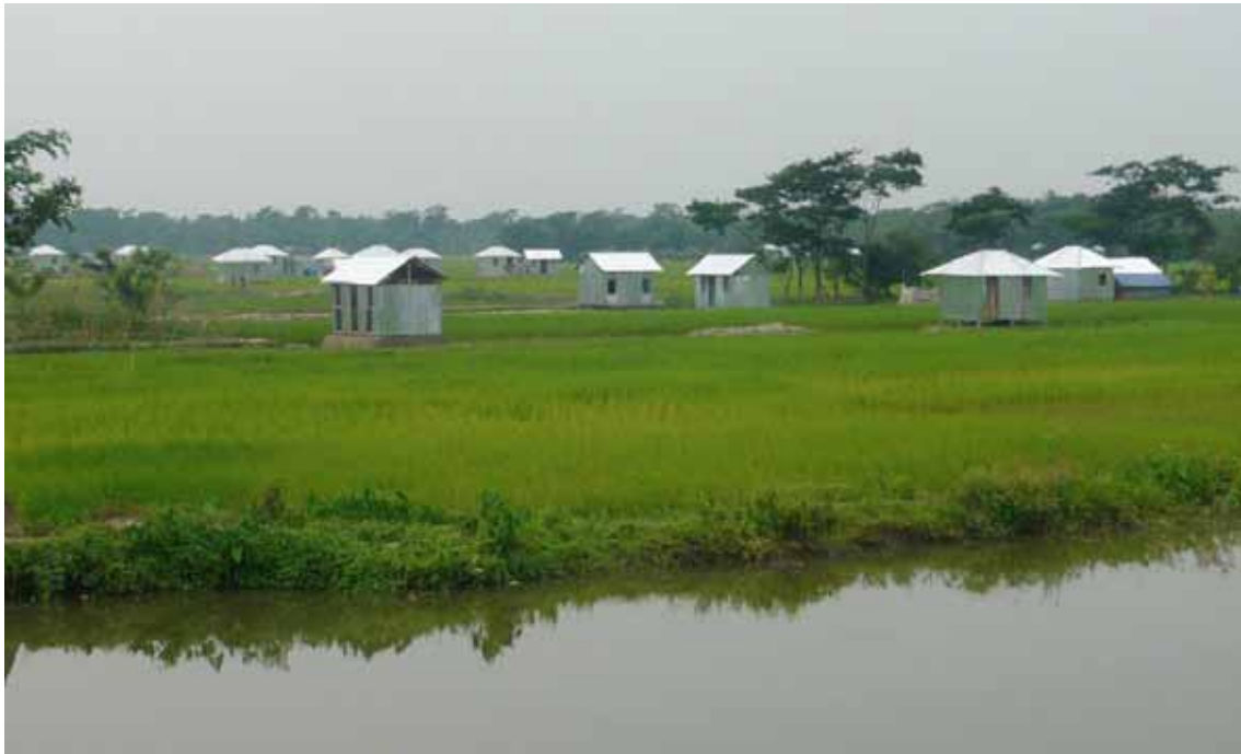
Figure 1. Construction of houses after the cyclone Sidr 2007.
