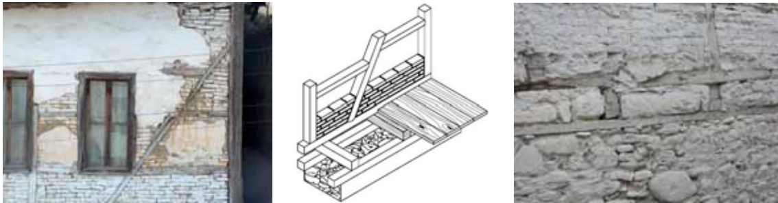
Figure 5: The Kalà di Elbasan (Albania), connection system
