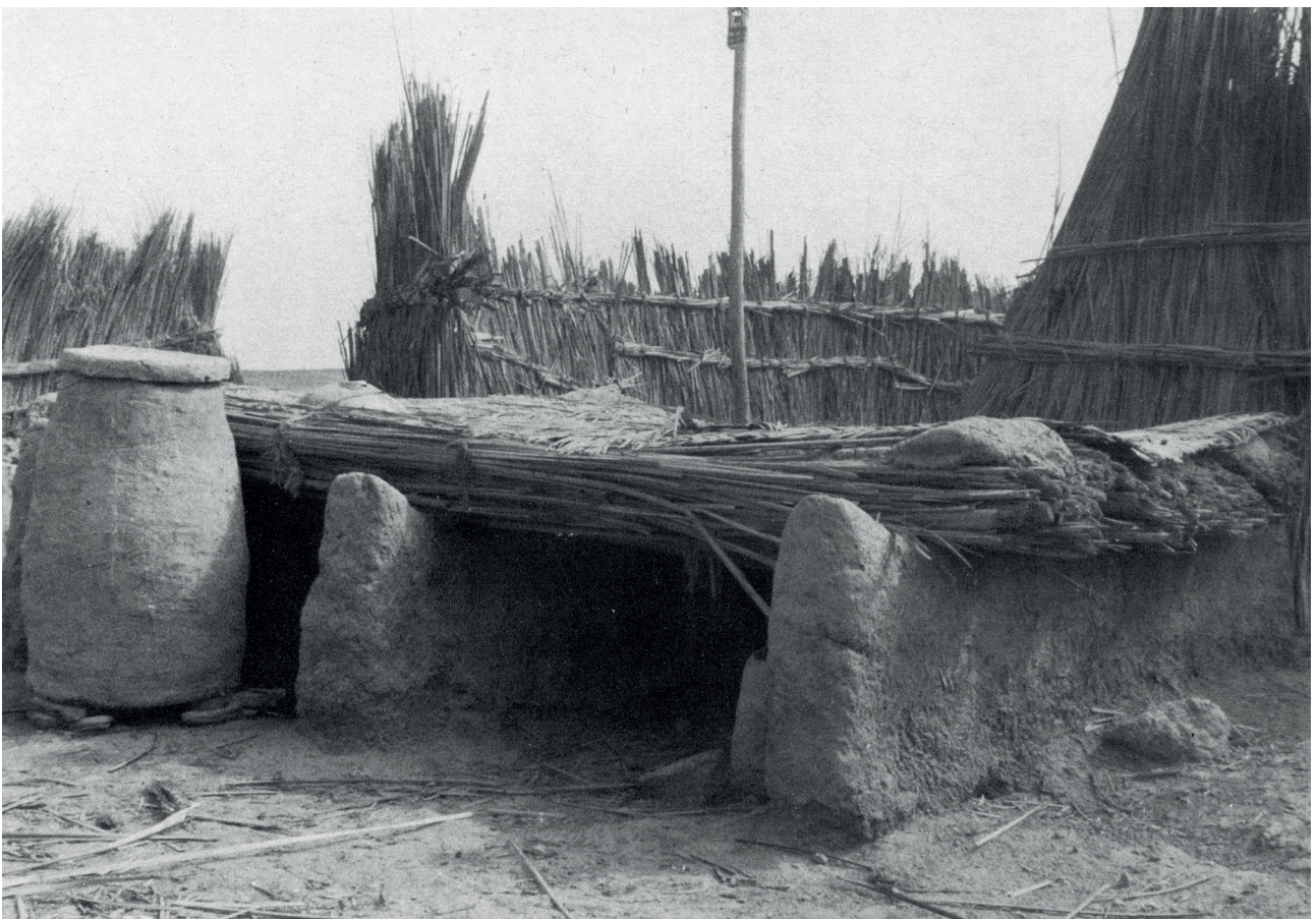
Fig. 1 – Bed built with mud and reeds, covered with a vegetal mat (Ochsenschlager, 1974, p. 172).
