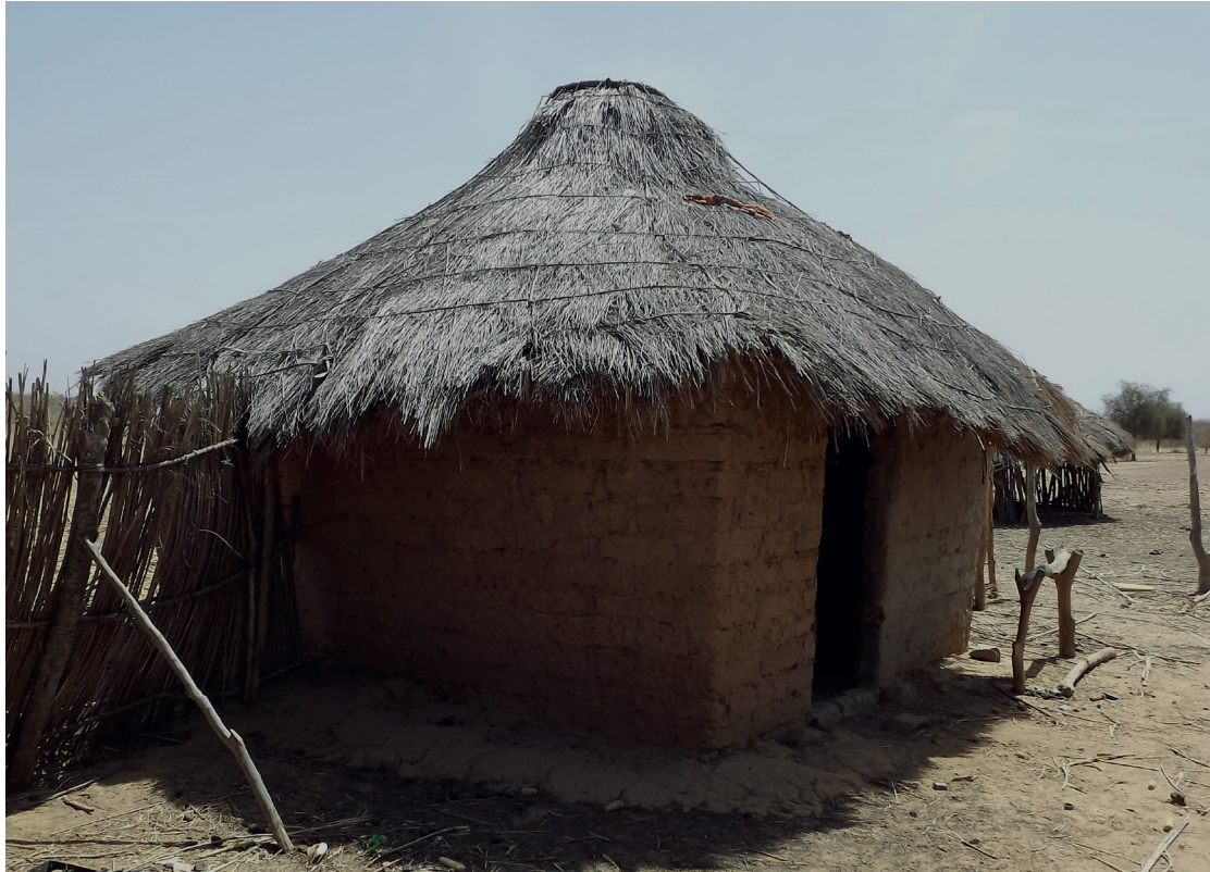
Fig. 6 – Habitation quadrangulaire H1 de la concession de Diabougou (cliché T. Pelmoine). Fig. 6 – Quadrangular dwelling H1 to the Diabougou compound (photo T. Pelmoine).
