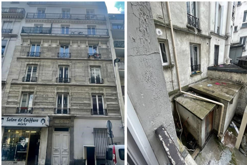
Figure 4. Building facade and view of the courtyard from inside an apartment.
