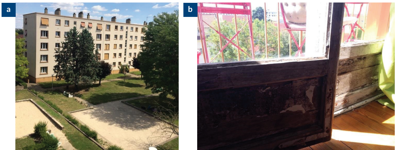
Figure 6. Current building photos (a) and windows from the interior (b).
