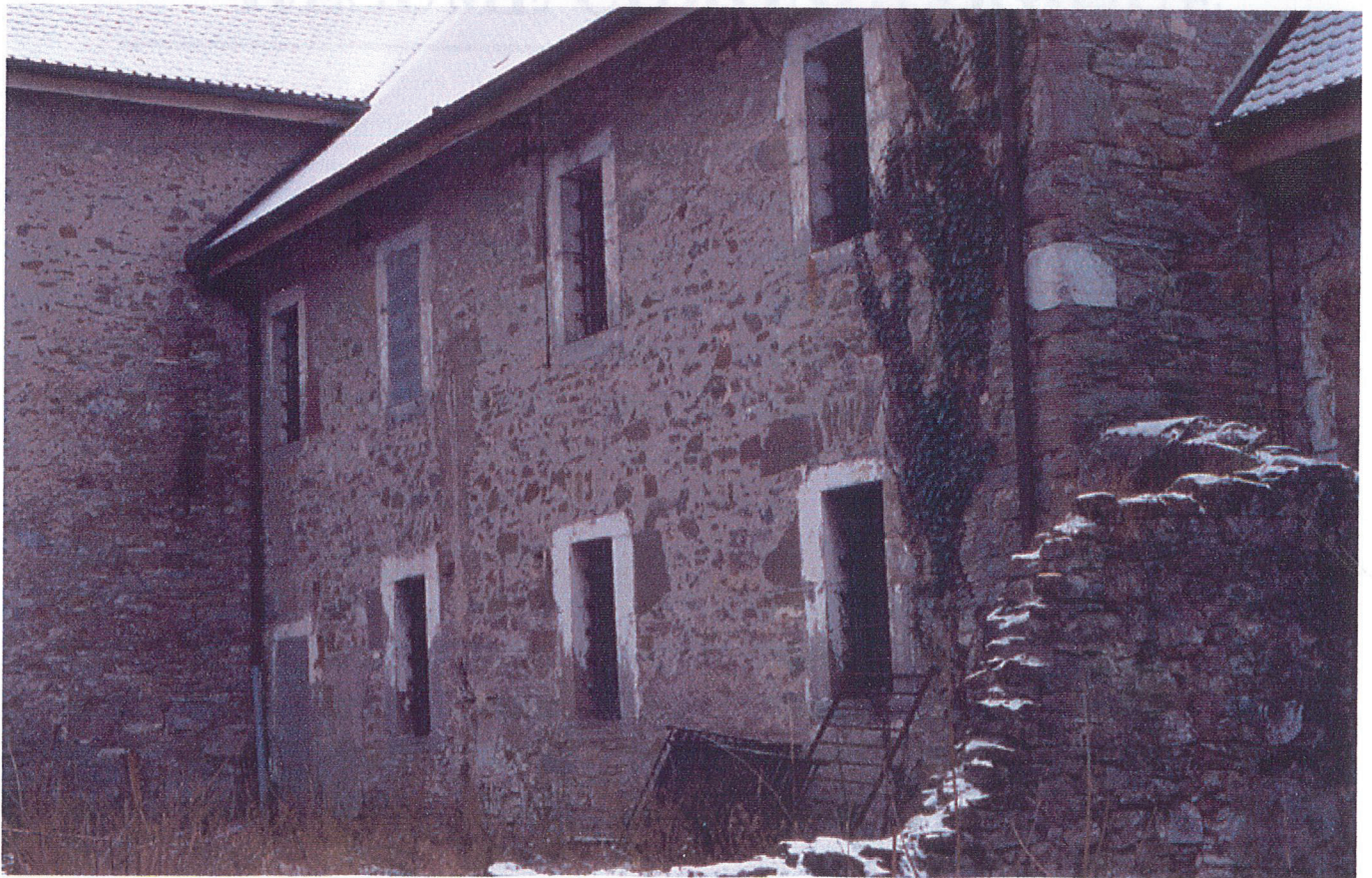
prison est, façade nord
