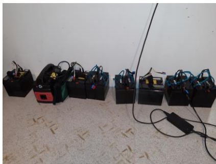
Figure 11: the necessary set of batteries required to complete a 1h mission for two UGVs
