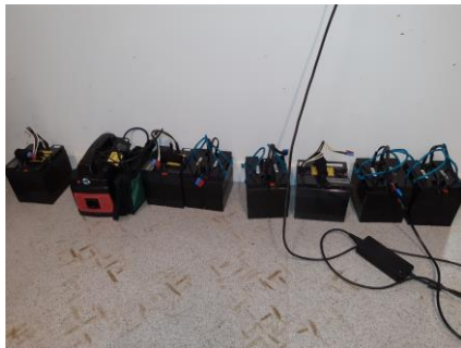
Figure 11: the necessary set of batteries required to complete a 1h mission for two UGVs
