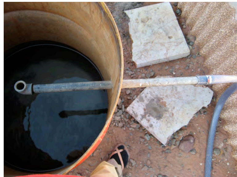
Water inlet metal pipe to flotation tank (without tap) 5
