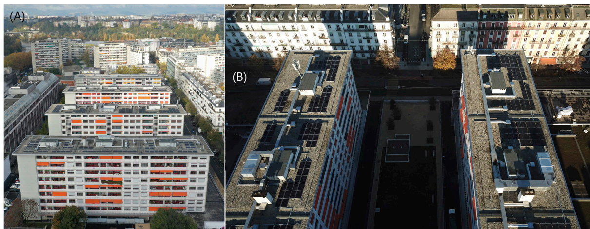
FIGURE 7 Completed renovation of the buildings (A), solar installation on the roofs with a limited area available due to technical equipment (B), published with the permission from © Hospice General Geneva.
